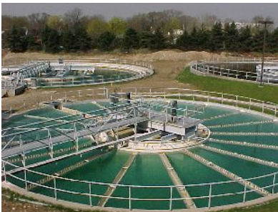
The water treatment system
